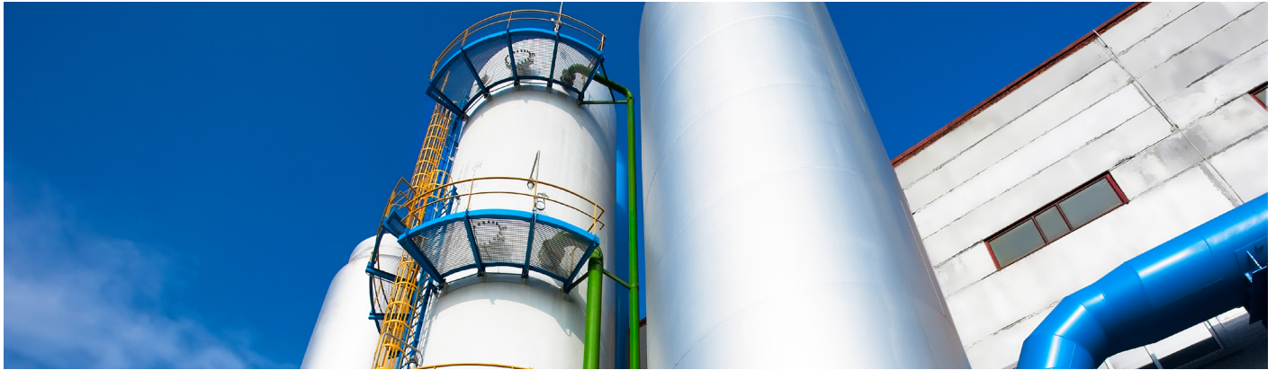
Air Separation Plant
