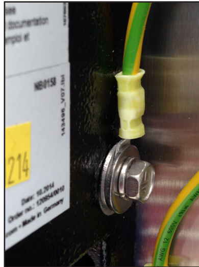
Figure 3 Earth Bolt And Nut Washer Assembly
