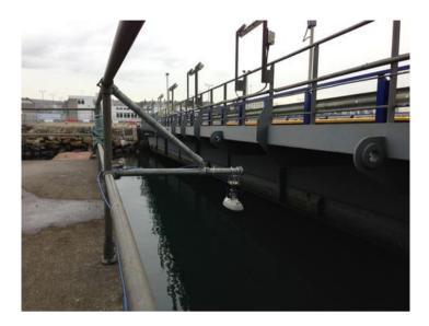
See example of boom constructed from standard scaffolding parts and attached to existing railing structure
