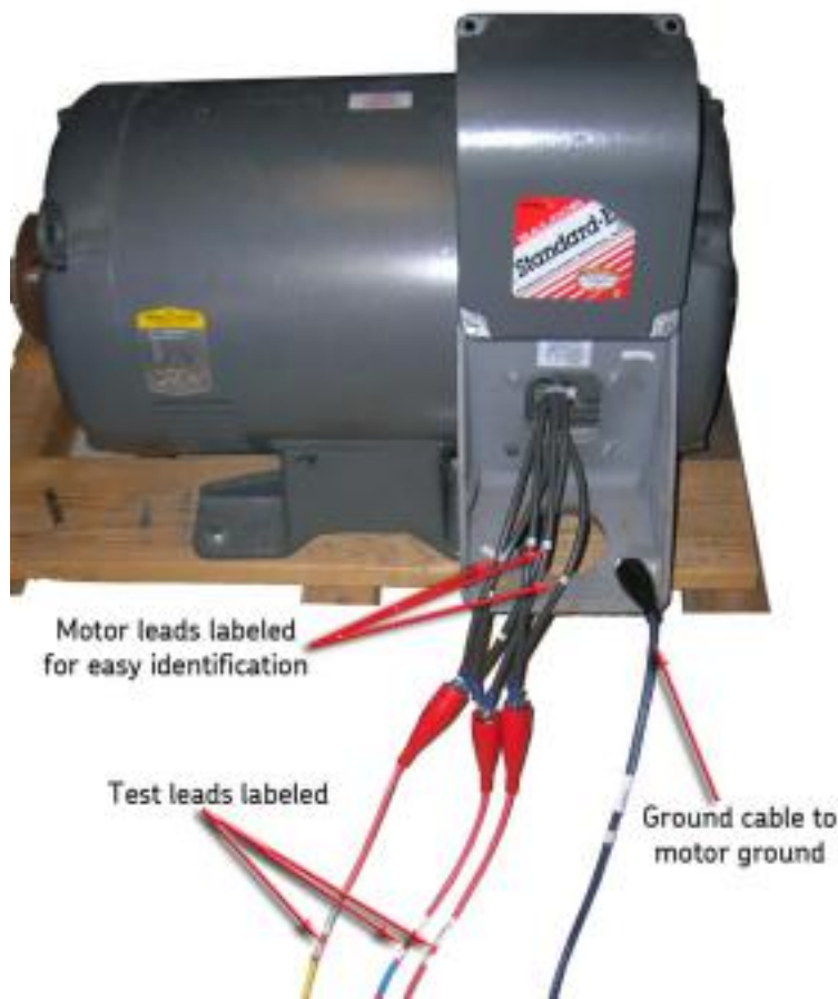
Figure 68. Connecting high-voltage test leads to motor leads.
